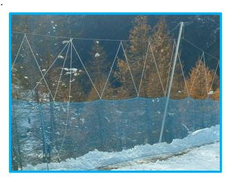
**A – NET** – The number of nets depends on the length, the meshes and thickness.
