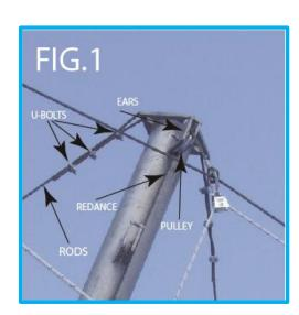
3) Mount at the top of the pole on the lateral holes, the rods blocking the cables with a minimum of three u-bolts. (Fig.1)
