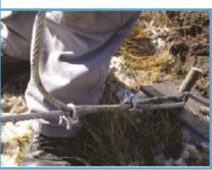
8) Value the pole rotation. After that, insert 4 pickets at the base with the hammer, then secure them in the ground.
